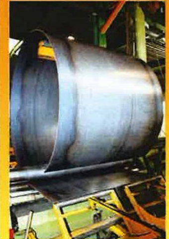
Tank rolling in progress
